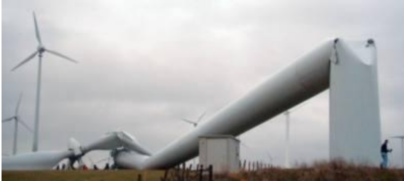
Turbine Structural failure in Western Germany
