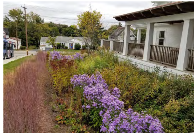
This rain garden at Mass Audubon's Broad Meadow Brook Wildlife Sanctuary is composed of native shrubs and flowers. It will temporarily hold stormwater runoff from the surrounding landscape and release it gradually.
