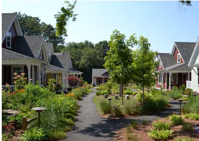
This Low Impact Development at Concord Riverwalk emphasizes less pavement and more green areas.
